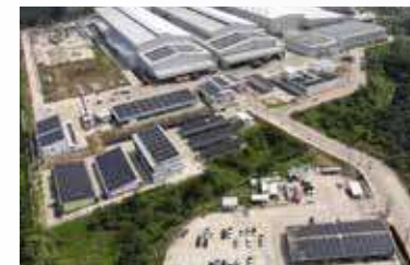
Solar rooftop at factory's Chumphon Branch
