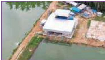
1. Location of Reclaim Water System
