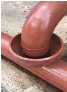
Water Collection Points for System
