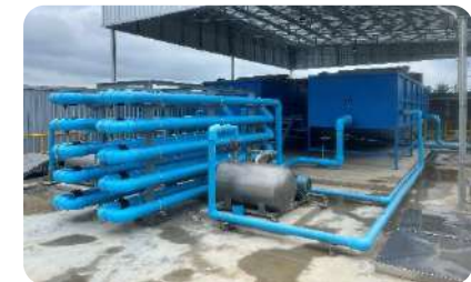
2. DAF Dissolved Air Flotation System
